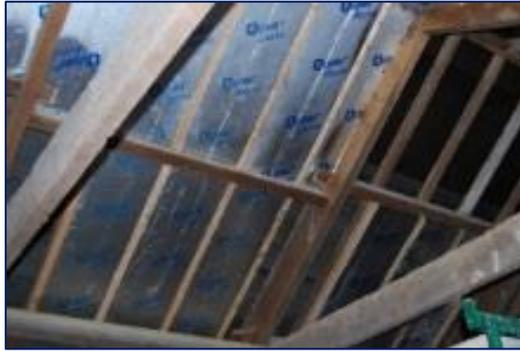
Figure 8: Typical roof insulation
