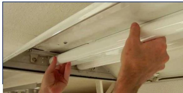
Figure 4: Removing individual lamps
